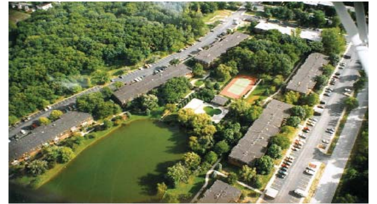
Aerial view of Mansards North in the mid 1970s.
