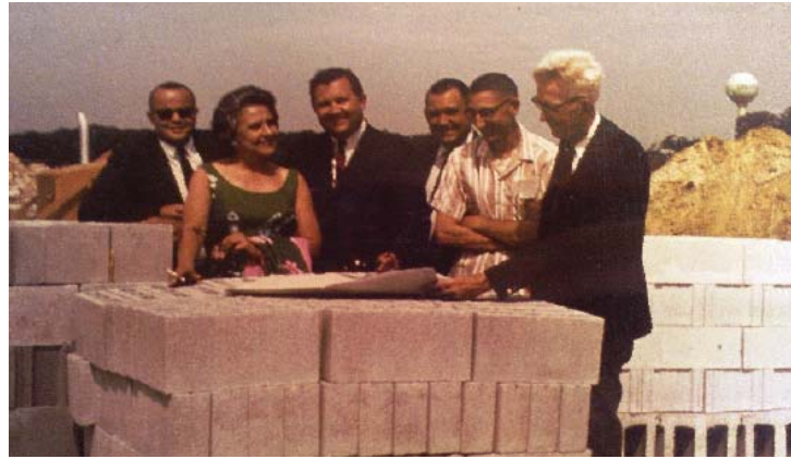
Building developers and Town of Griffith officials on the construction site at the North side of The Mansards.
